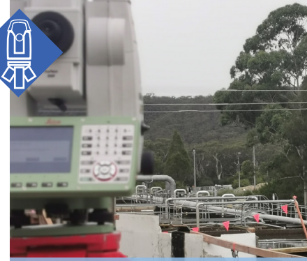
Wastewater Treatment Plant Upgrade
