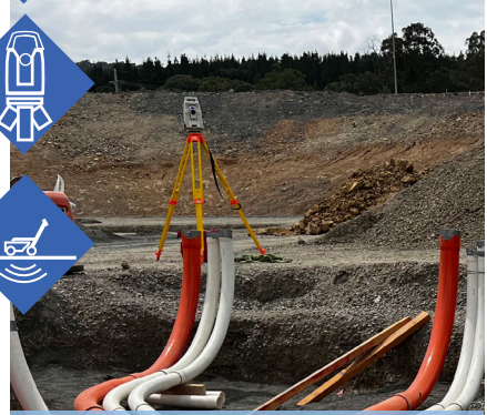
Cadia Ventilation Fans VR11 & VR51
