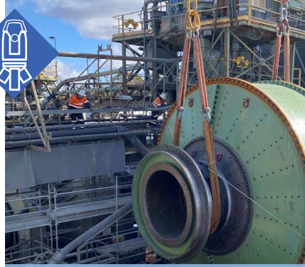
Cobar Mine Replacement Mill
