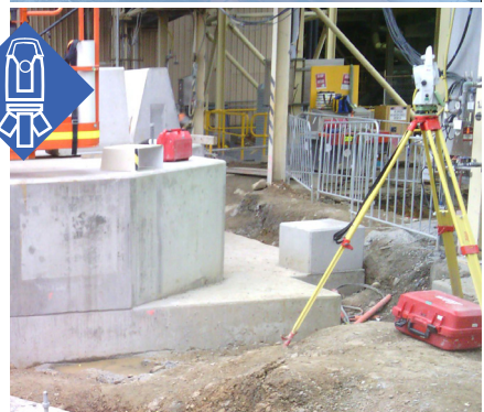
Cadia Expansion Project Stage 1 Civil & SMP
