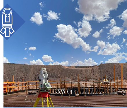
Prominent Hill Shaft Collars & Civil
