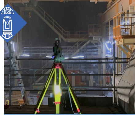
Cadia U/G Expansion Project
