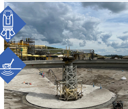
Cadia Expansion Project Stage 2 Civil
